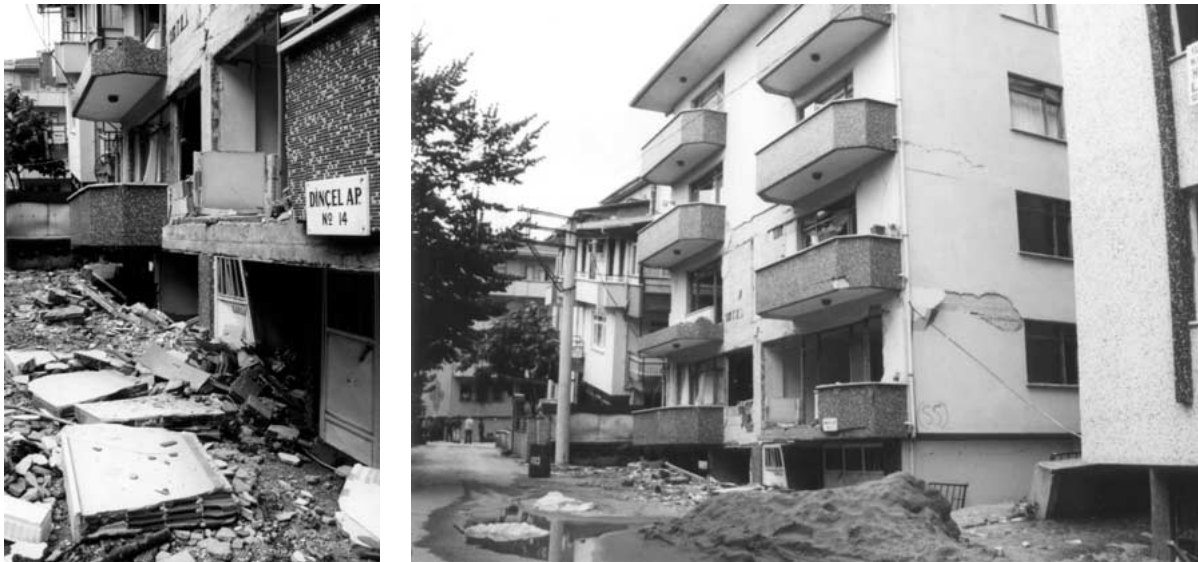
Figure 1. Damage due to foundation failure.
