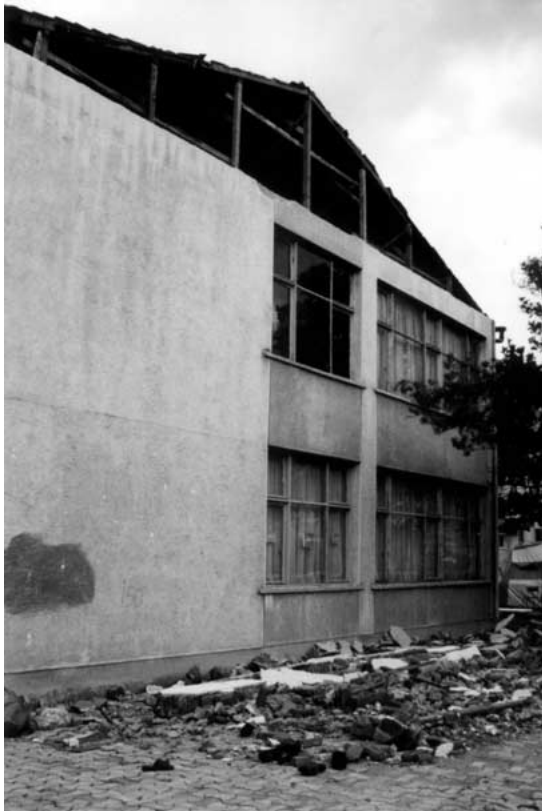
Figure 25. Nonstructural damage to a school building.
