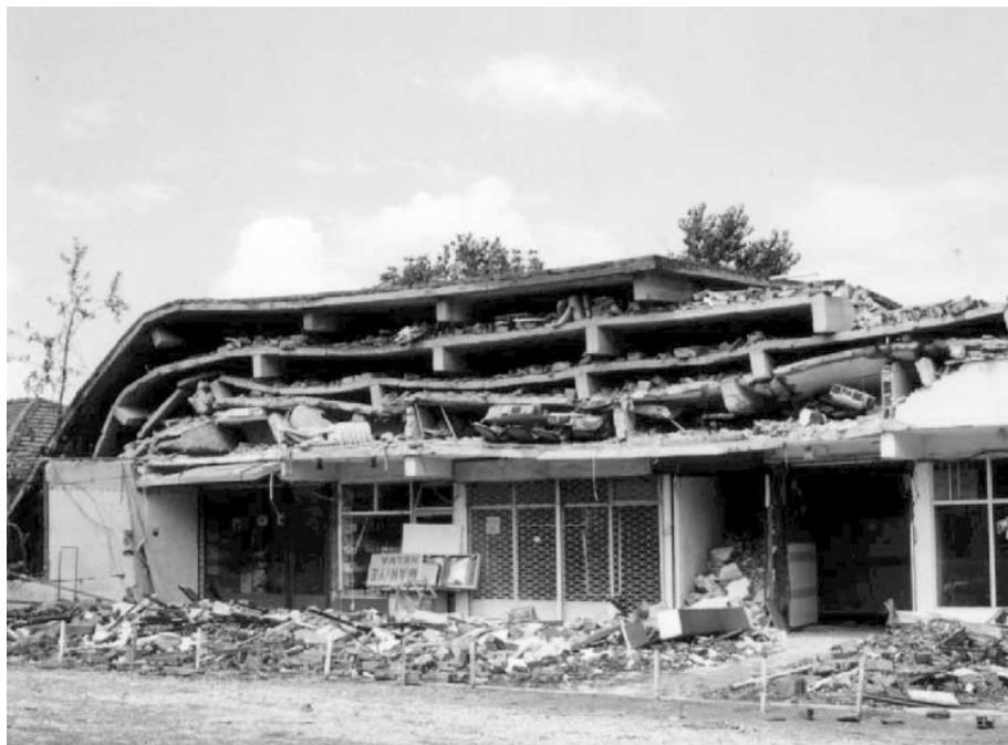
Figure 27. Typical building adjacent to retrofitted Sakarya 'province' government building.
