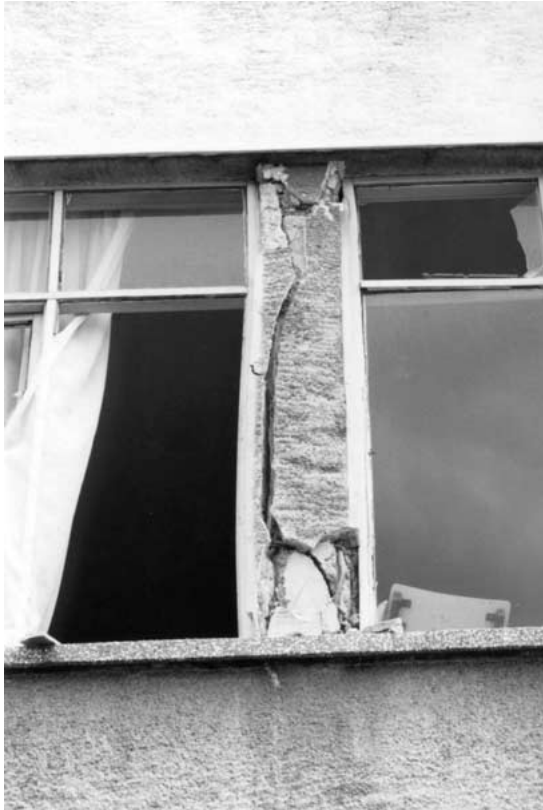
Figure 15. Damage due to flexural failure in non-ductile plastic hinges.
