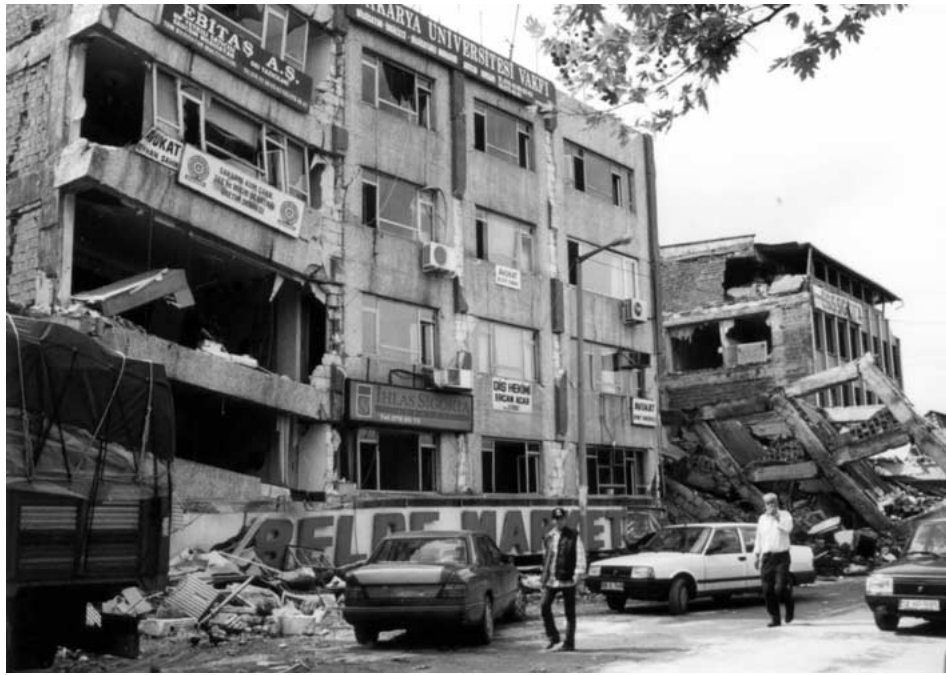
Figure 6. Failure of the soft first story.
