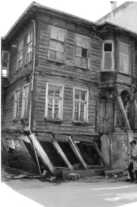
Figure 5. Failure of the soft first story in a timber building.
