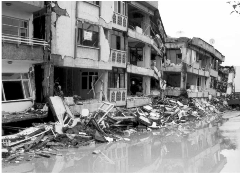
Figure 7. Failure of the soft first story.
