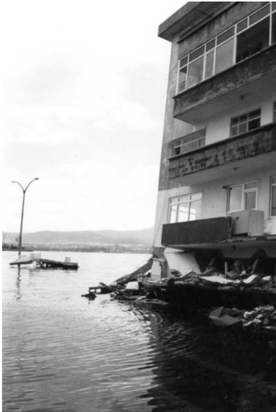
Figure 11. Some waterfront buildings were impacted by both geotechnical and structural failures.
