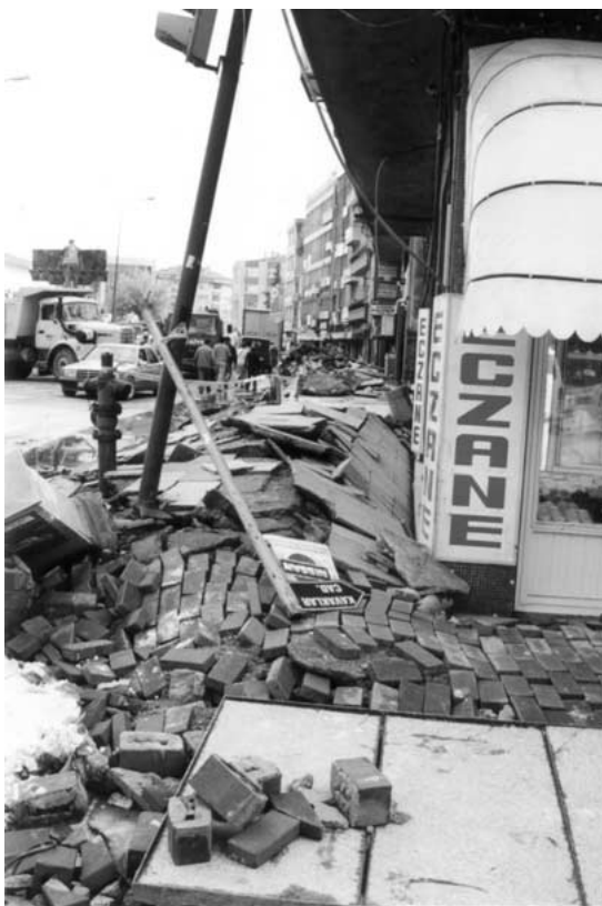
Figure 2. Ground heave was extensive all around this building.
