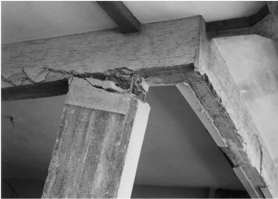
Figure 18. Example of bar pull-out due to deficient anchorage.
