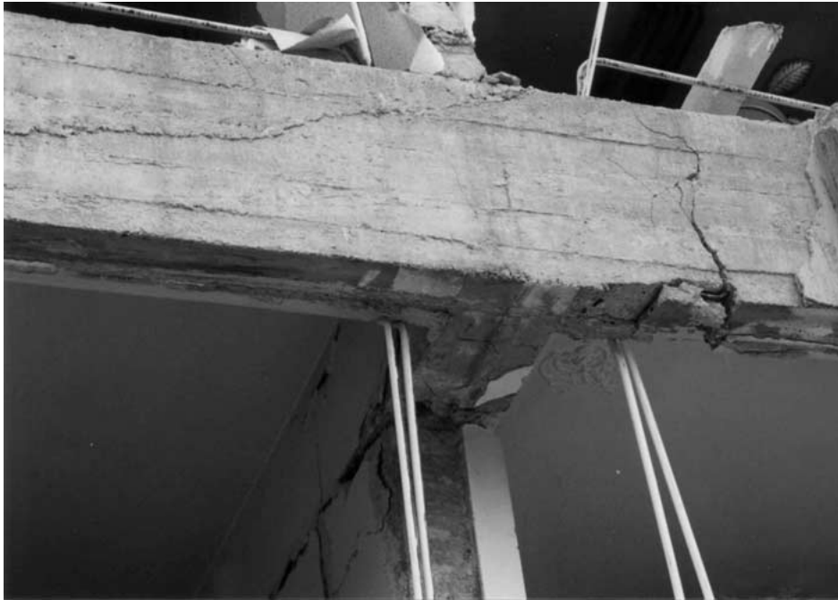
Figure 16. Damage due to eccentric beam-to-column connections.
