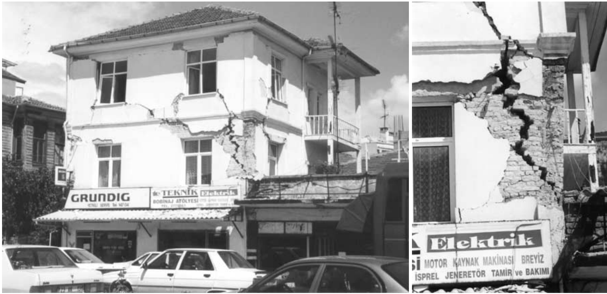
Figure 24. Damage to an unreinforced masonry building.
