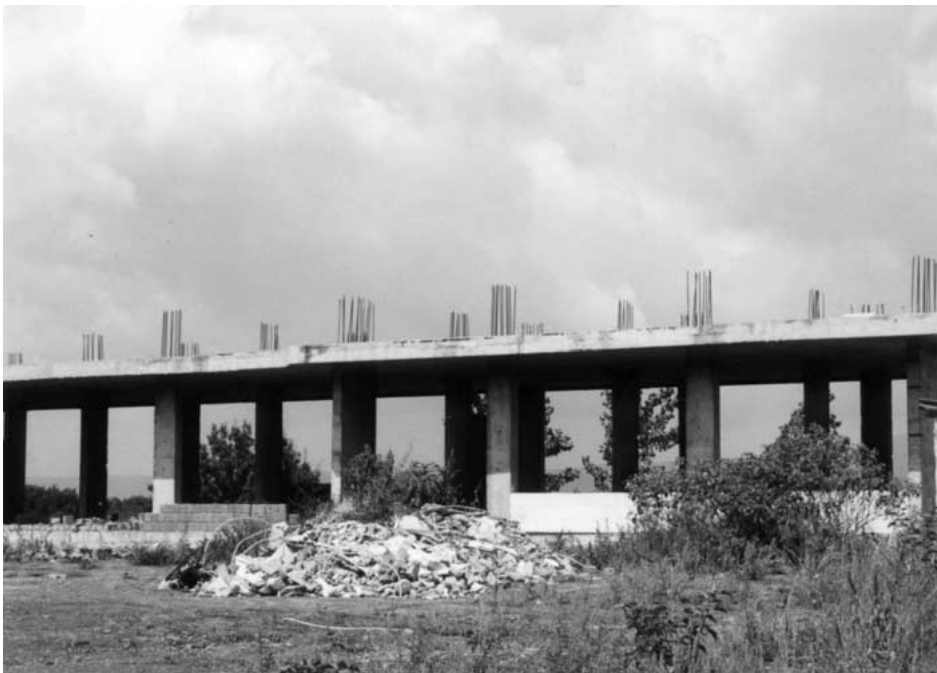
Figure 17. One story building during construction with column bars extended above roof slab to accommodate possible construction of other stories in future years.
