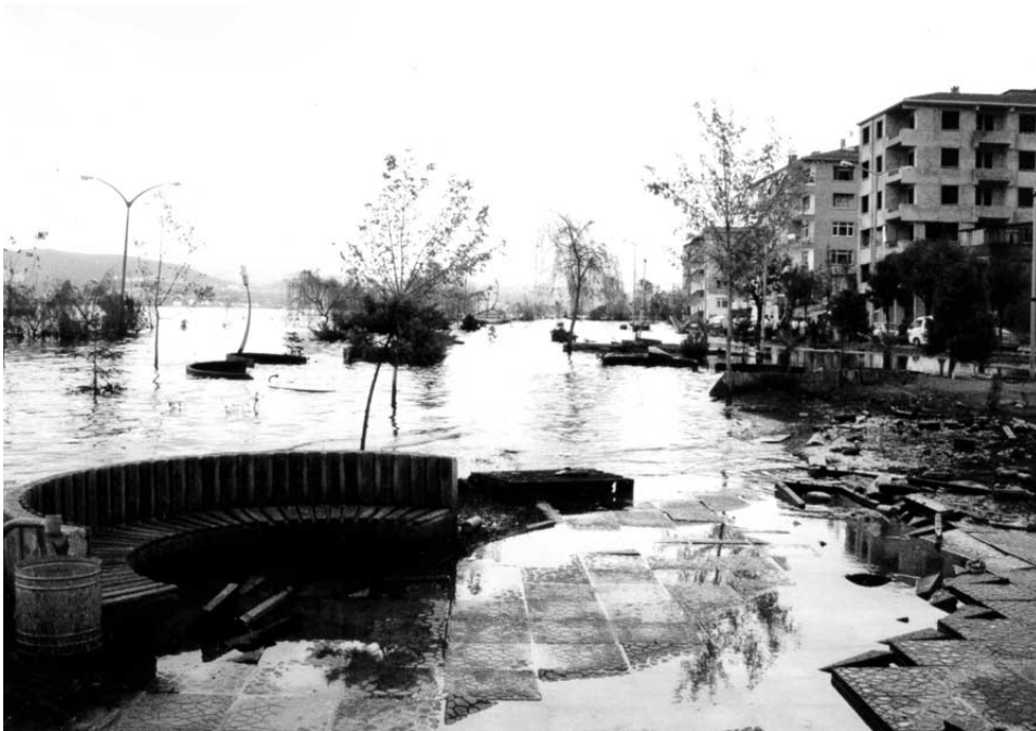
Figure 10. Marmara Sea submerged parts of the waterfront as a result of ground lateral spreading.
