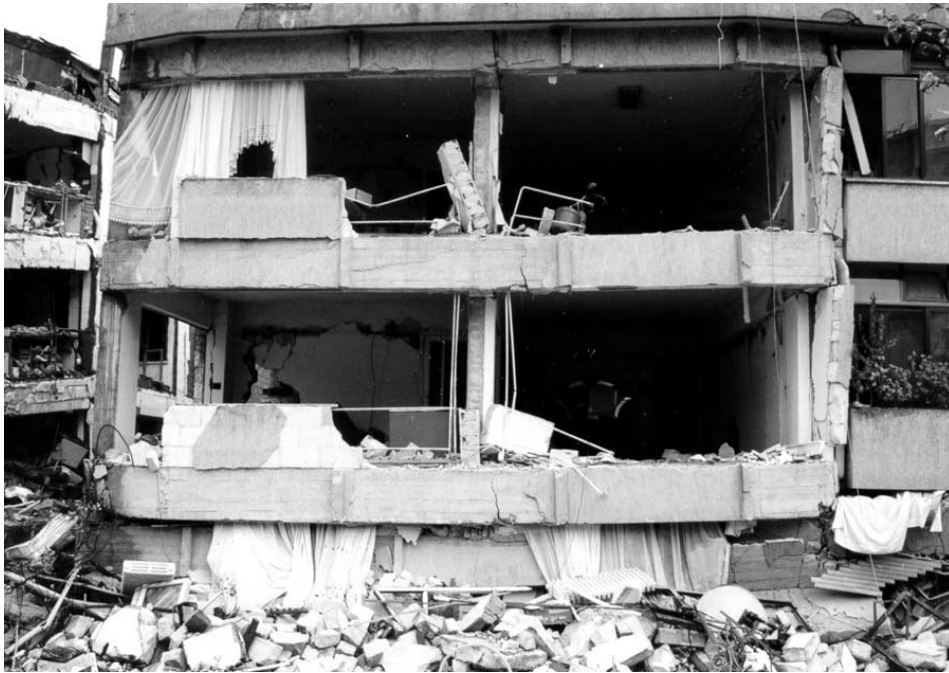
Figure 13. Damage due to strong beams and weak columns.
