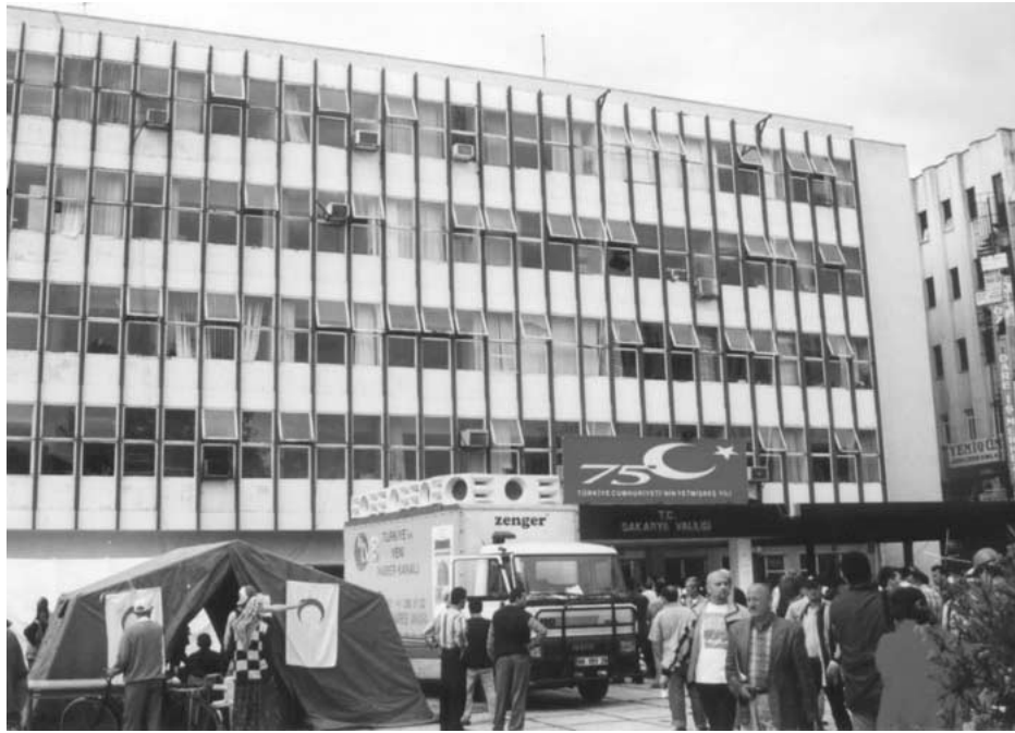
Figure 26. Undamaged Sakarya 'province' government building retrofitted by shear walls prior to earthquake.
