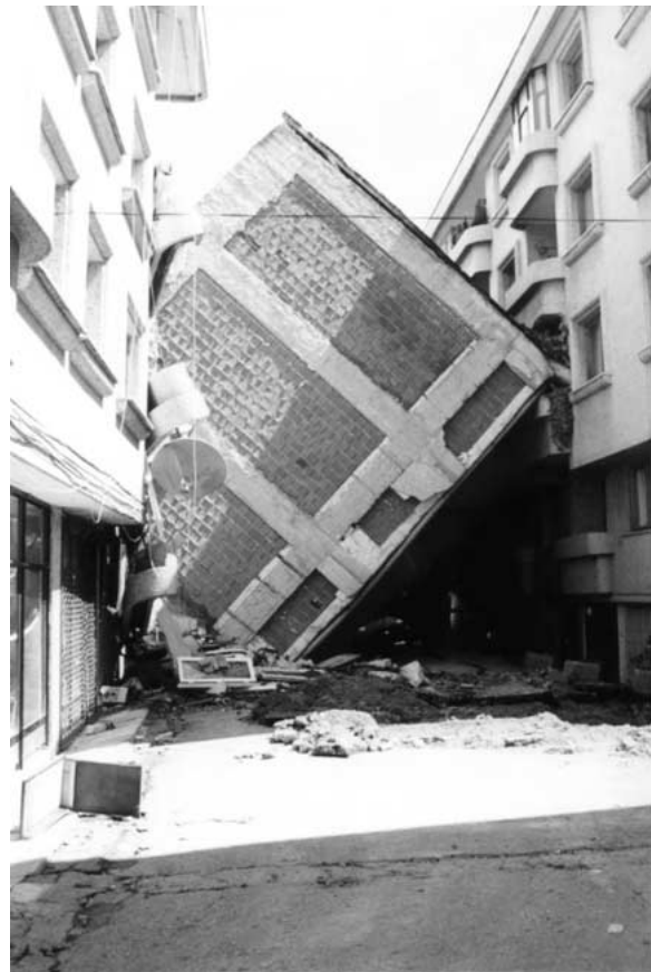
Figure 8. Failure of the soft first story.
