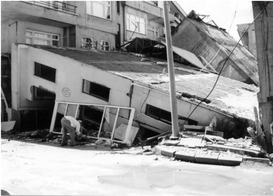
Figure 3. Overturned building due to foundation failure.
