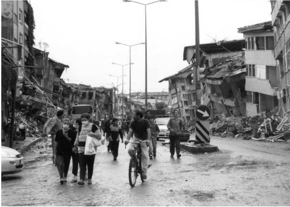
Figure 9. Buildings in this commercial area collapsed towards the street due to open facades (soft story) and walls on back side adding torsional eccentricity.
