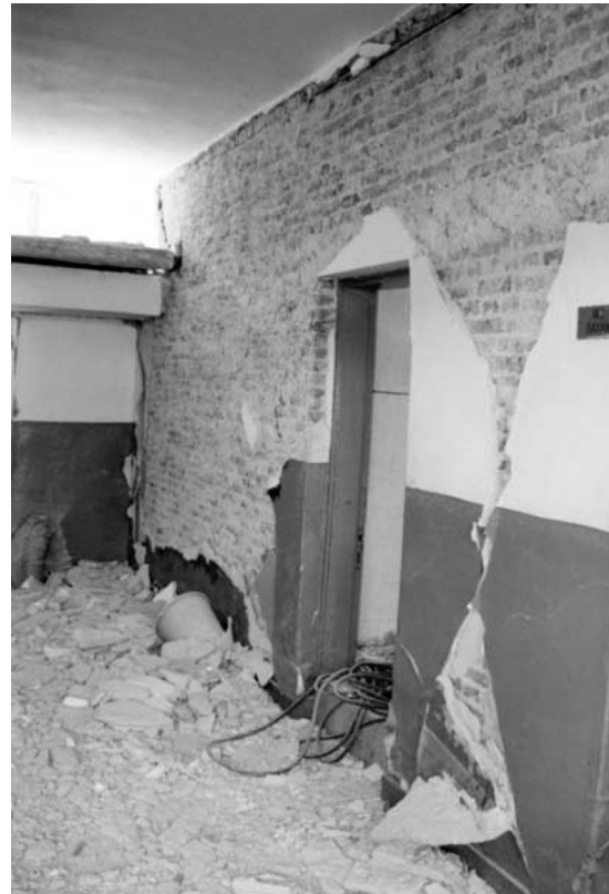
Figure 25. Nonstructural damage to a school building.
