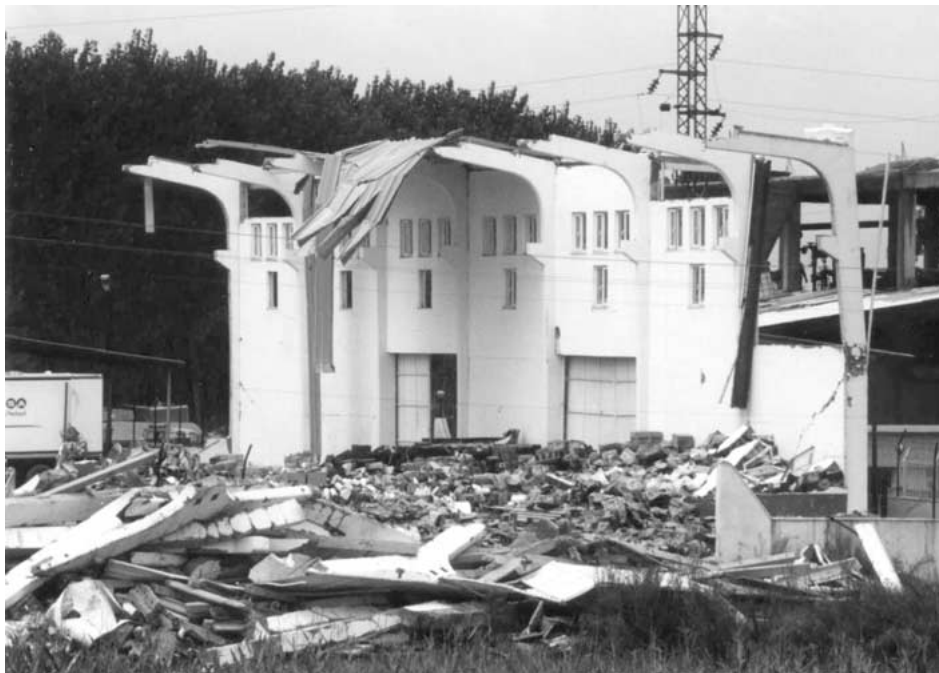
Figure 23. Damage to a precast concrete building.
