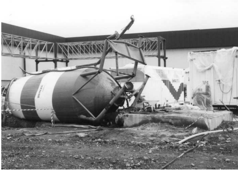
Figure 22. Overturned reservoir.
